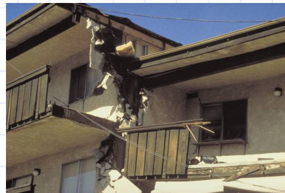
Northridge Meadows Apartment Complex
